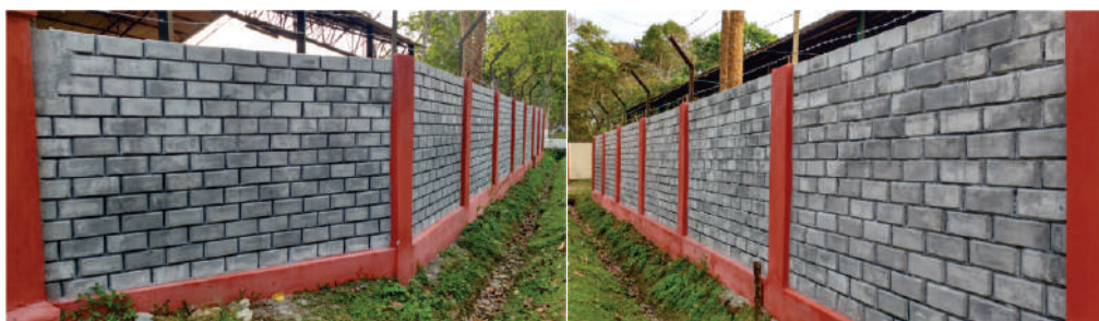
Constructed wall at CSIR-NEIST premise using Modular bricks
